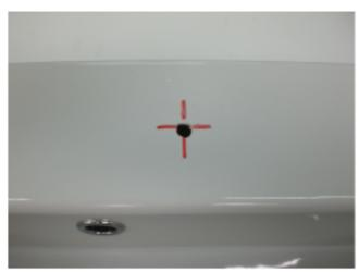
Continue to strike until a small hole is created in the upper part while in the lower part the ceramic disc has completely cleared.
