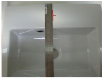
On the upper level of the tap mark the centre of the hole from the rear of wash-hand basin as taken from the measurement on the technical specification.
